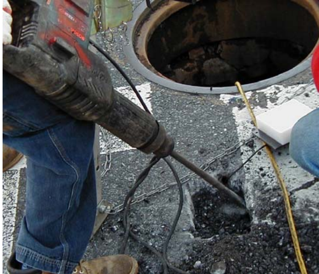
Figure 3: Chipping out the antenna recess
