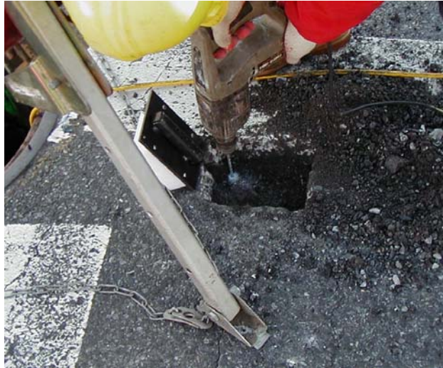
Figure 5: Drilling holes for wedge anchors
